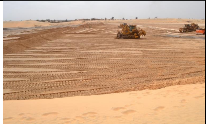
Figure 5: Reprofilage
