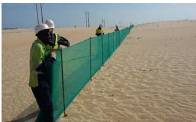
Figure 33 & 34. Installation de filets brise-vents
