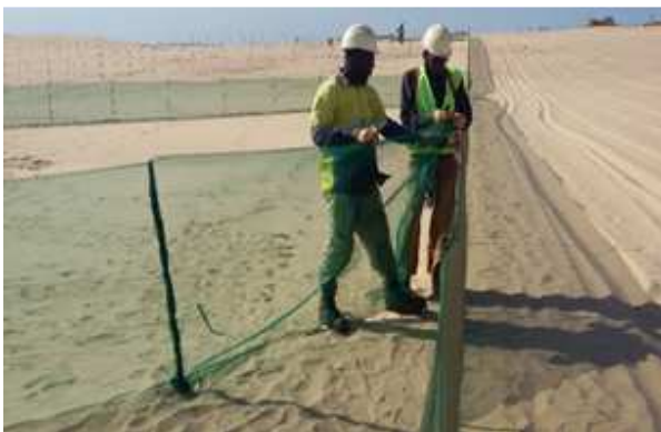
Figure 25. Installation de filets brise-vents
