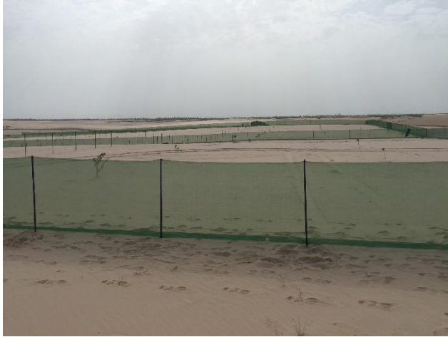
Figure 24. Installation de filets brise-vents
